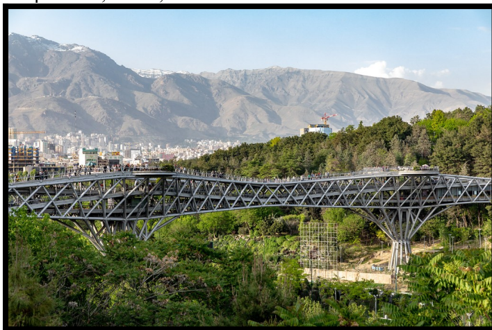
Fig. 6. Tabiat Bridge in Tehran (2014)
